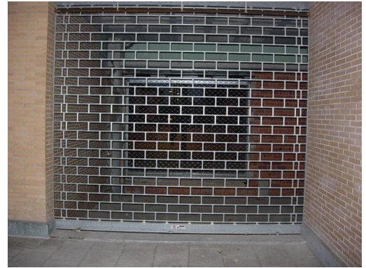
| CONNECTING PIECE ** Steel flat bar, plastic stop and end caps.
